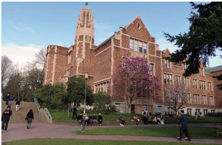
The Music Building has been a beloved and highly recognizable structure on the UW's north campus since 1950. Planned improvements will help the School of Music better serve its students, faculty, and UW community now and into the future.
